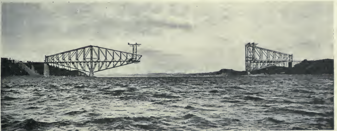
Fig. 1.—General view of Quebec Bridge to date—showing erection progress to the end of the season, 1915.
